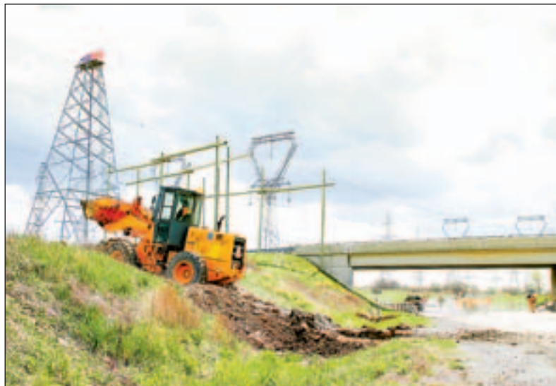
Cleanup crews move in to take away barriers erected Friday.
